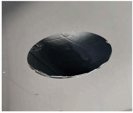
Put register into retaining ring, and felt ring on top.
